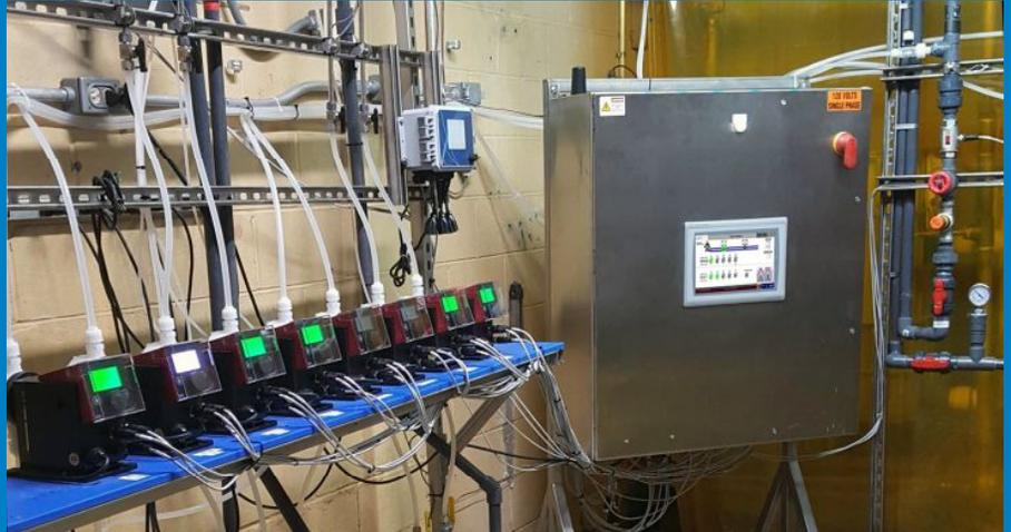
“Introducing a PLC-based control system and a custom algorithm for this poultry processor’s flow-based chemical feed and monitoring system saved product, system downtime, and significantly reduced USDA violations.”
