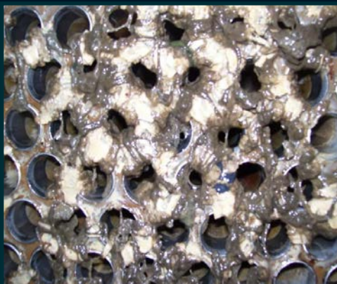
(June 2008) U15 Main Condenser Tube Sheet after extended run – before cleaning, after non- MIOX treatment
